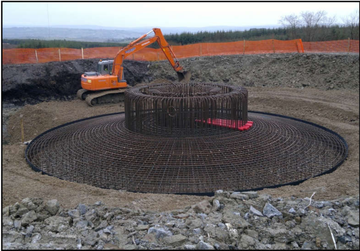
Figure 4-24: Construction of a wind turbine base
