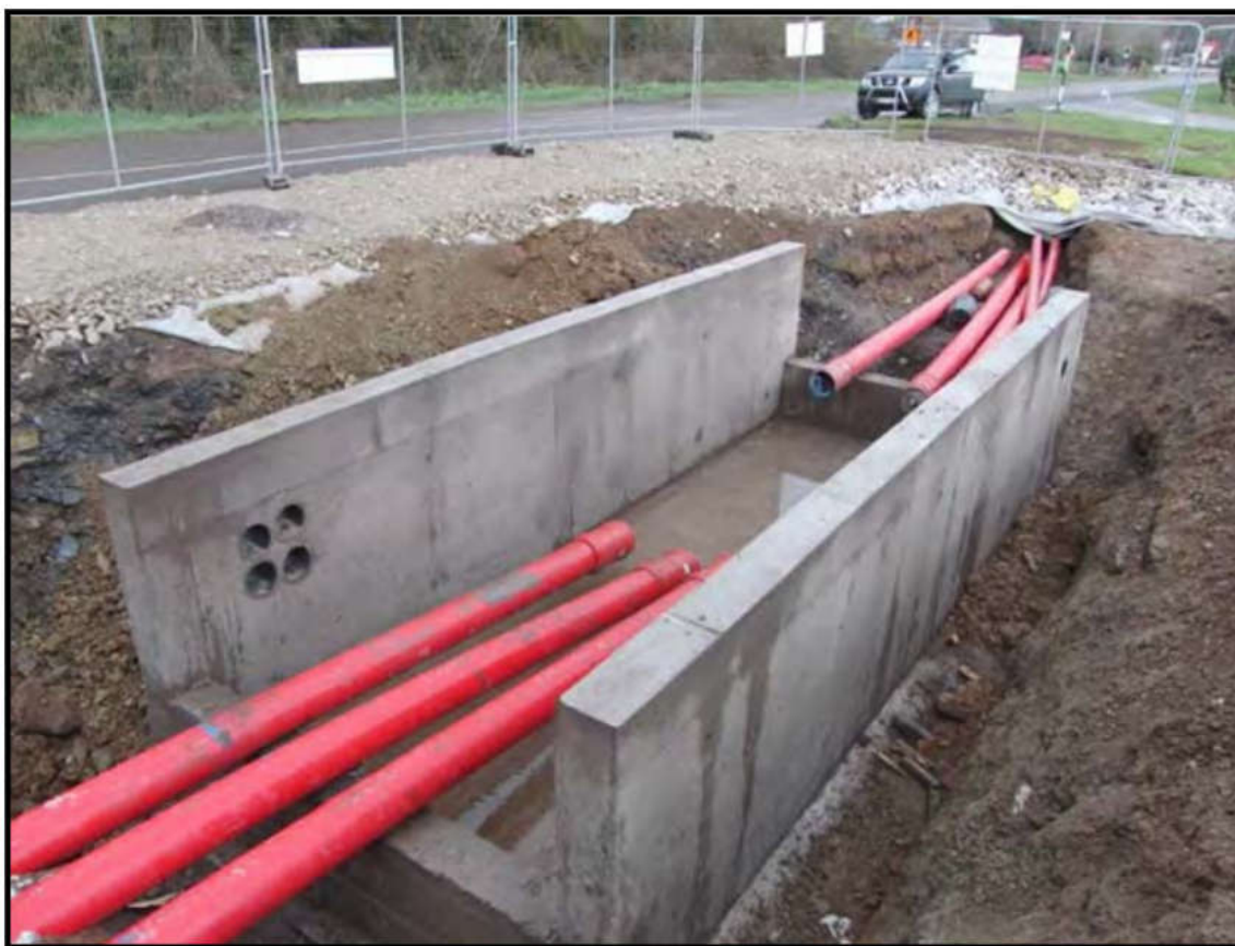
Figure 4-32: A joint bay construction
