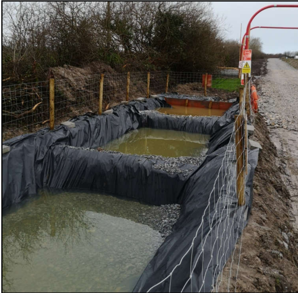
Figure 4-20: A Multi-tiered settlement pond with stone filter
