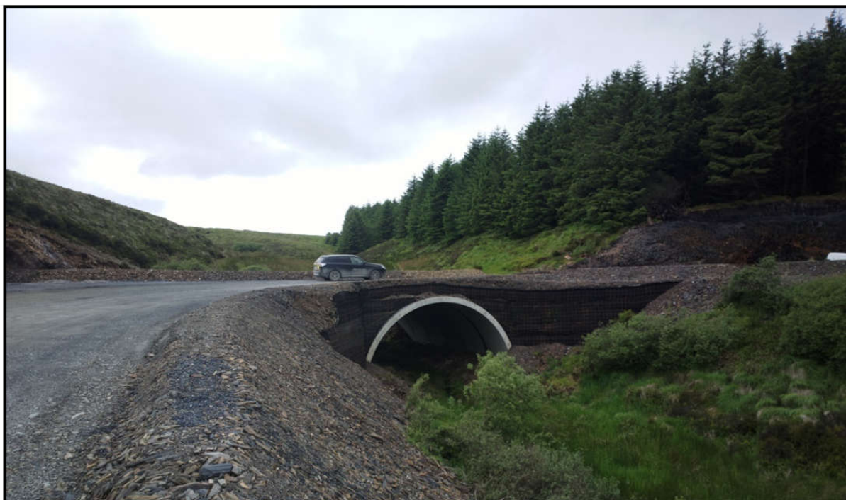
Figure 4-15: Completed clear span pre-cast concrete culvert crossing over existing watercourse
