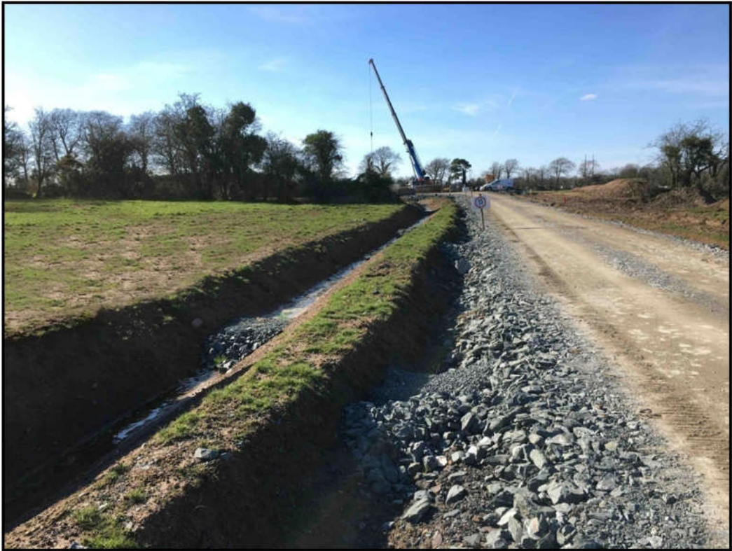
Figure 4-12: Separation of Clean and Dirty Water Drainage on a Wind Farm Site
