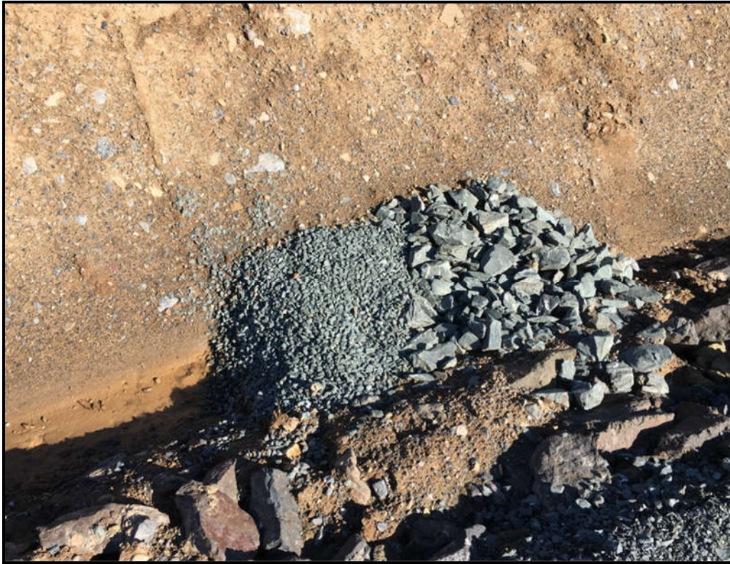
Figure 4-19: A stone check dam with large aggregate on downstream side
