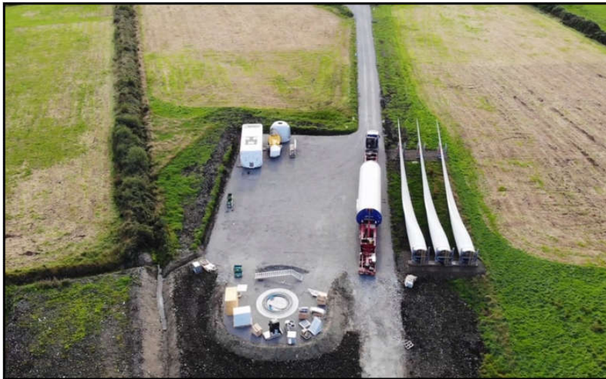
Figure 4-23: A finished hardstand on a wind farm
