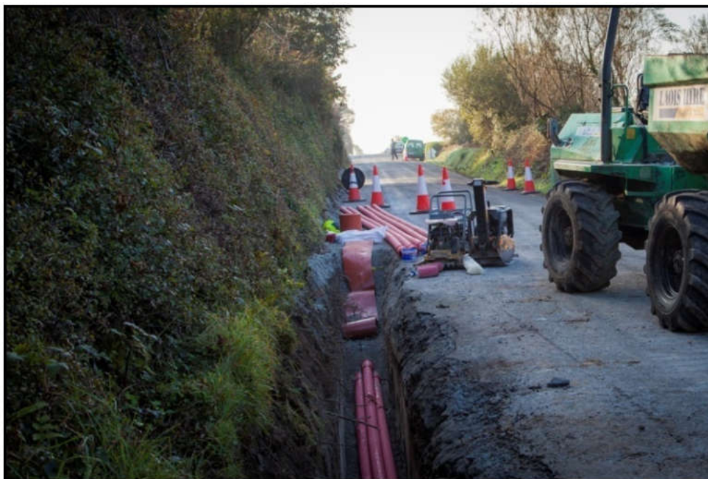
Figure 4-27: Ducting installation works for a grid connection cable trench
