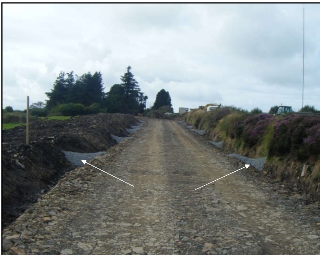
Figure 4-21: Check dams along roadside drainage channels
